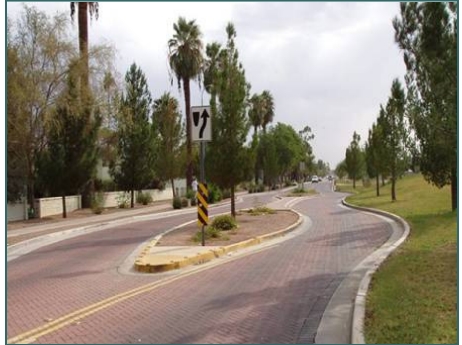
Permanent Traffic Islands on 48th Street south of Indian School Road
